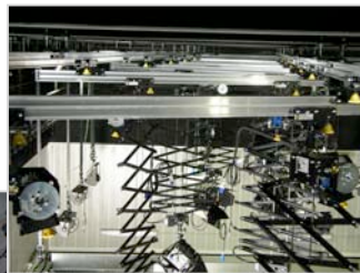
AL RAY Studio 4 - KUWAIT TYPICAL COLD LIGHTING DMX CONTROLLED (CST FRESNELS & FLUORESCENTS) INSTALLATION, USING THE "D" RAIL WITH INTEGRATED DMX AND MAINS ELECTRICAL DISTRIBUTION
